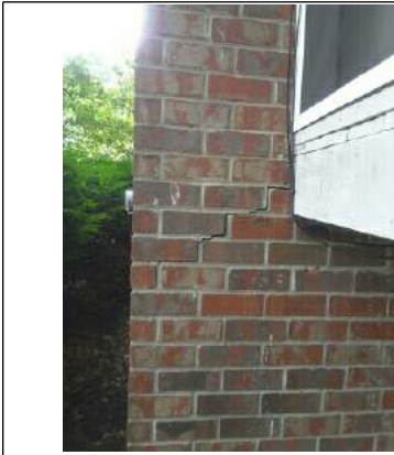
Northeast wall step cracks. This is by the deck on the corner. The block on the other side in the crawlspace had step cracks also.
