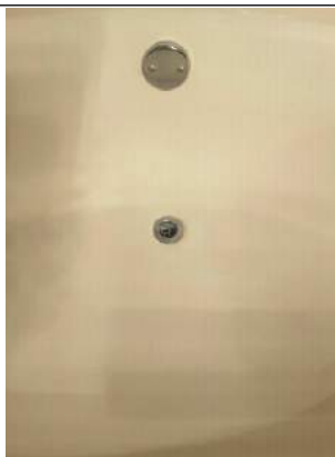
Missing drain plug in tub.
